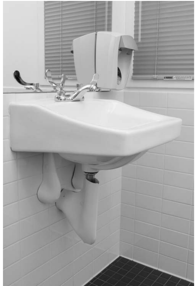
Figure 25-23 Insulating the hot water pipes and drain under a sink prevents burns to the lower extremities of wheelchair users.
