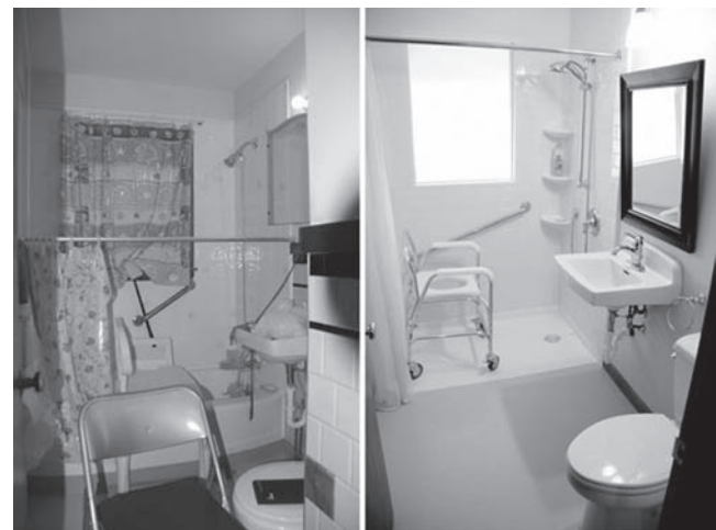
Figure 31-1 The photo on the left is a typical bathroom with sink, toilet, and shower. A grab bar and a tub transfer bench are in the shower to assist with transfers. The wall-hung sink without a cabinet is accessible to roll under. The pipe is insulated to prevent leg burns. The transfer bench prohibits the shower curtain from fully closing and water gets on the floor. The lighting is poor and the space is cluttered. The photo on the right has been modified and has a curbless shower with a handheld shower head. The rolling bath seat allows for transfer prior to reaching the shower. The cutout in the seat allows for washing without having to stand. The lighting is improved with access to natural lighting as well as ambient lighting. Clutter has been removed. (Photos courtesy of Lifewise Renovations, Prairie Village, KS.)
