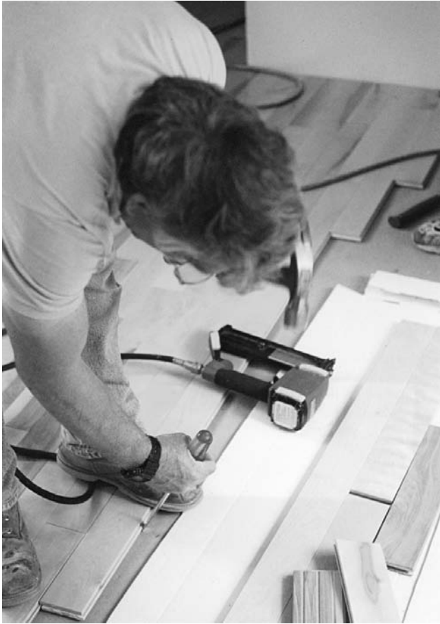
Figure 1-6 Self-advancement role: contractor; task: installing floor; activity: moving the wood into place.
