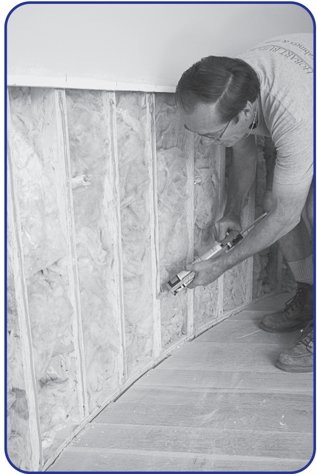
FIGURE 65.2 Don using a caulking gun.
