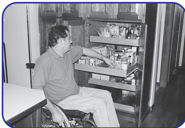
FIGURE 46.14 Shallow drawers on gliders make all goods accessible from a seated position.
