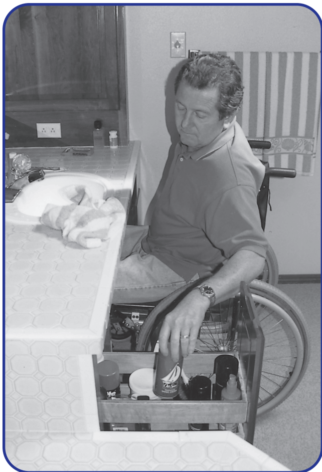
FIGURE 46.12 Recessed plumbing and double-deep drawers allow easy access to the sink area from a seated position.
