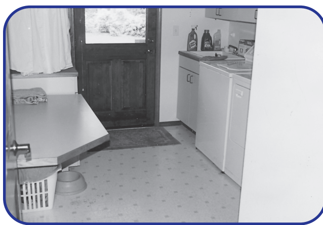
FIGURE 46.16 The laundry table is angled to allow a clear pathway for the wheelchair, and the counter height is 32 in. for ease of use when seated, with clear access underneath.
