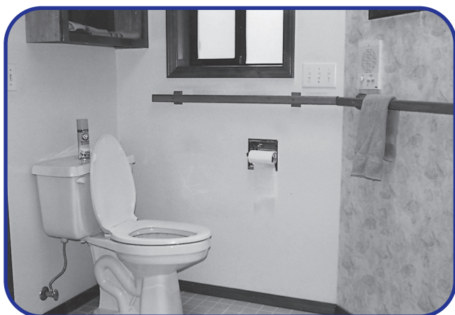
FIGURE 46.13 The oak grab bars also serve as a towel rack and the extra-high toilet enables an easy side-to-side transfer from a wheelchair.
